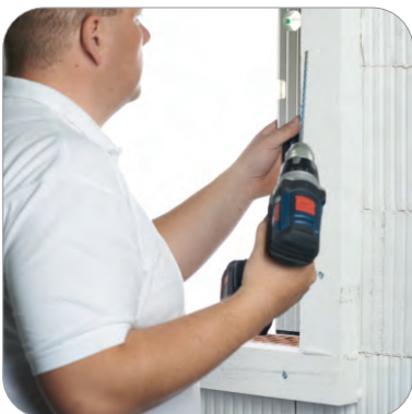
Side greenteQ Climate Conformal Profiles Align greenteQ Climate Conformal Profiles with the perpendicular and secure using greenteQ Window Frame Screws Flat Head
