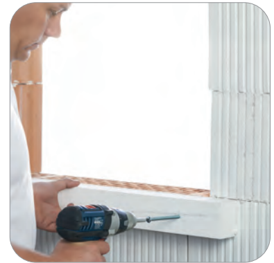
Lower greenteQ Climate Conformal Profile Attach greenteQ Climate Conformal Profile on wall and secure using greenteQ Window Frame Screws Flat Head
