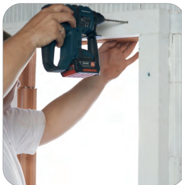
Upper greenteQ Climate Conformal Profile Attach greenteQ Climate Conformal Profile at top on side Climate Conformal Profiles and secure using greenteQ Window Frame Screws Flat Head
