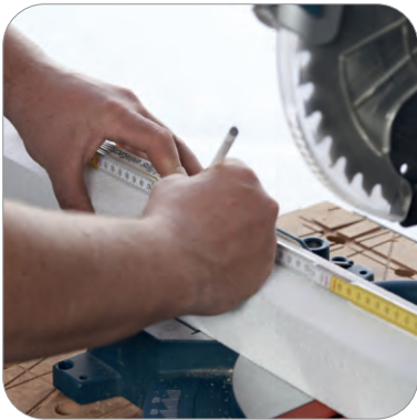
Measuring and cutting the greenteQ Climate Conformal Profiles to size Mark the respective dimension on the greenteQ Climate Conformal Profile and cut to size
