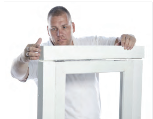
Preassembly of frame in case of external installation
